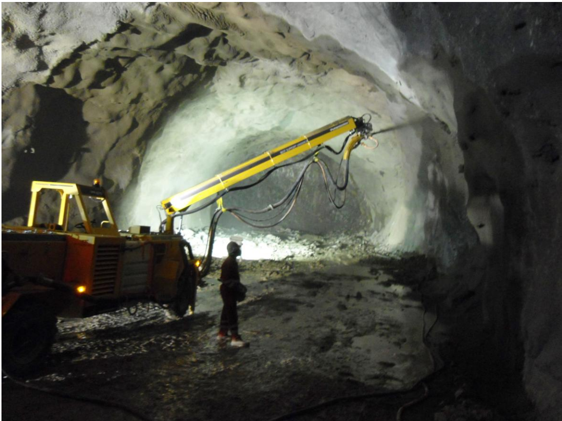
Photo: SPM 4210 WETKRET concrete spraying system at work
